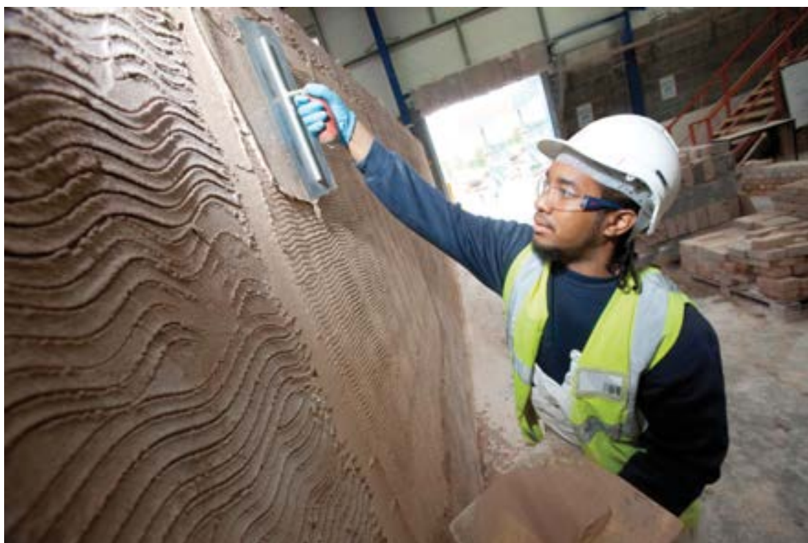
Matthew McAllastair is a plastering apprentice employed by Frank Haslam Milan (Keepmoat Group) and trained by CITB.
