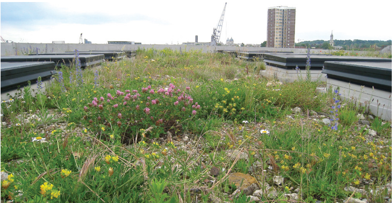
Laban Centre, Deptford. The green roof is constructed of crushed concrete from demolition material sourced from the site prior to construction.
