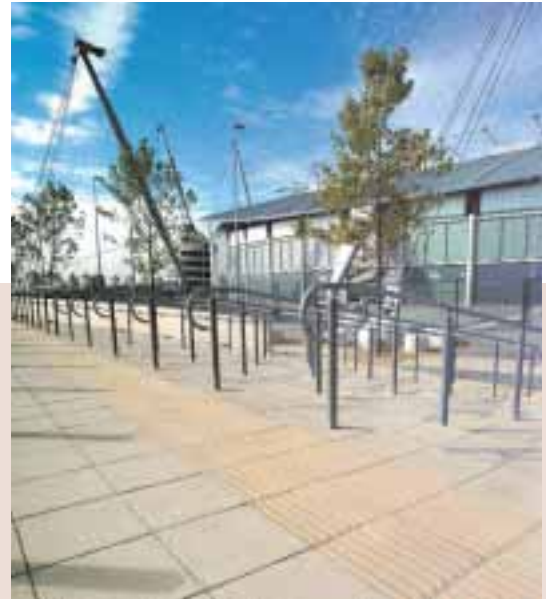
Hazard Warning Paving, City Stadium, Manchester
