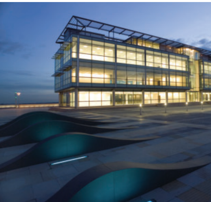
Island Wharf, Hull
