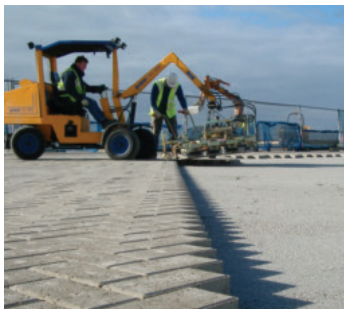
Machine lay of concrete block paving
