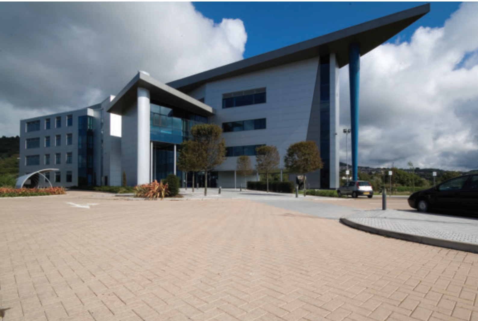
Keyblok and Stein & Design Pallas, Baglan Technium Building, West Glamorgan
