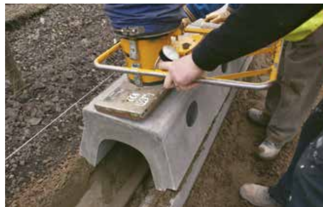
Beany Block installation, mechanically handled
