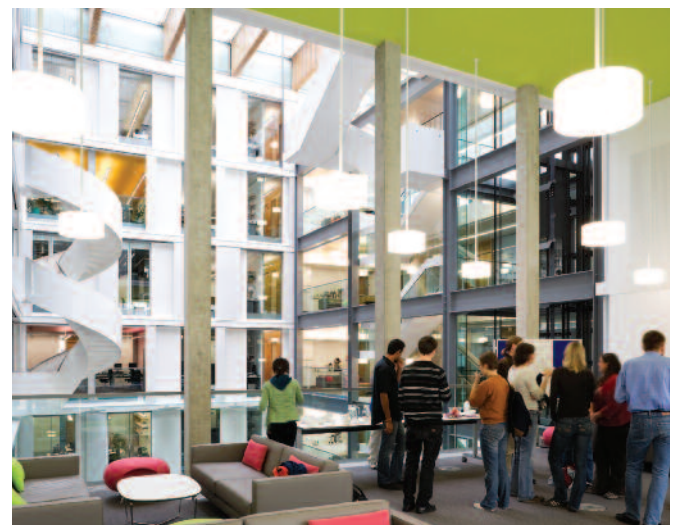
The Informatics Forum at Edinburgh University, designed by Bennetts Associates, has exposed concrete offering high thermal mass and has achieved a BREEAM rating of 'Excellent'.
