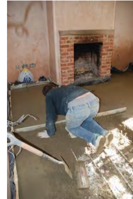
Labour Intensive Laying of Screed
