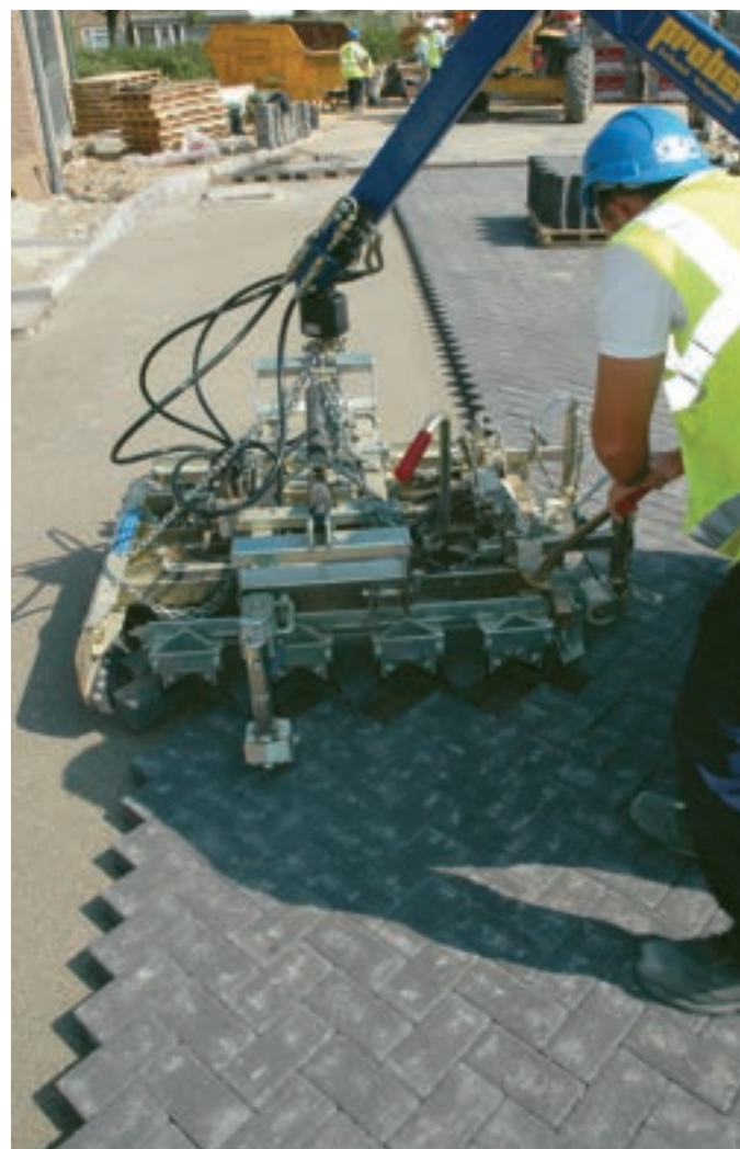
Installation of Marshalls ML Products
