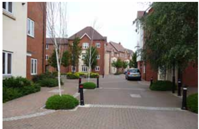
Permeable concrete and concrete block paving (shown above) can be used to reduce, attenuate and treat surface water as part of a sustainable drainage solution (SuDS). The water can then be used within the landscape to enhance biodiversity.
