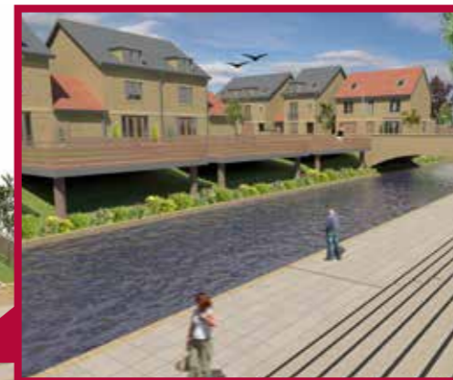
Linear channel into an attenuation pond
