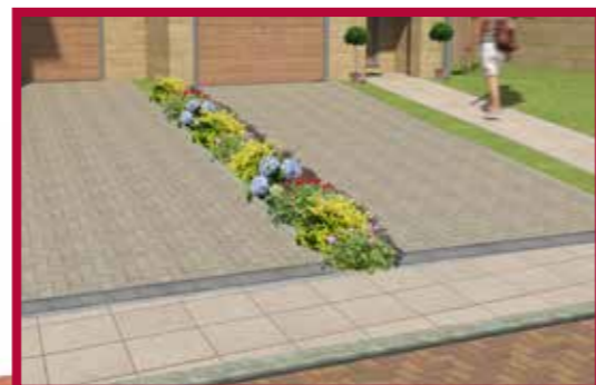
Linear drainage directed to a tree pit
